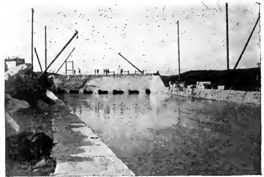
FIG. 4.—HEAD GATES, NEW CANAL, GARVIN'S FALLS.
